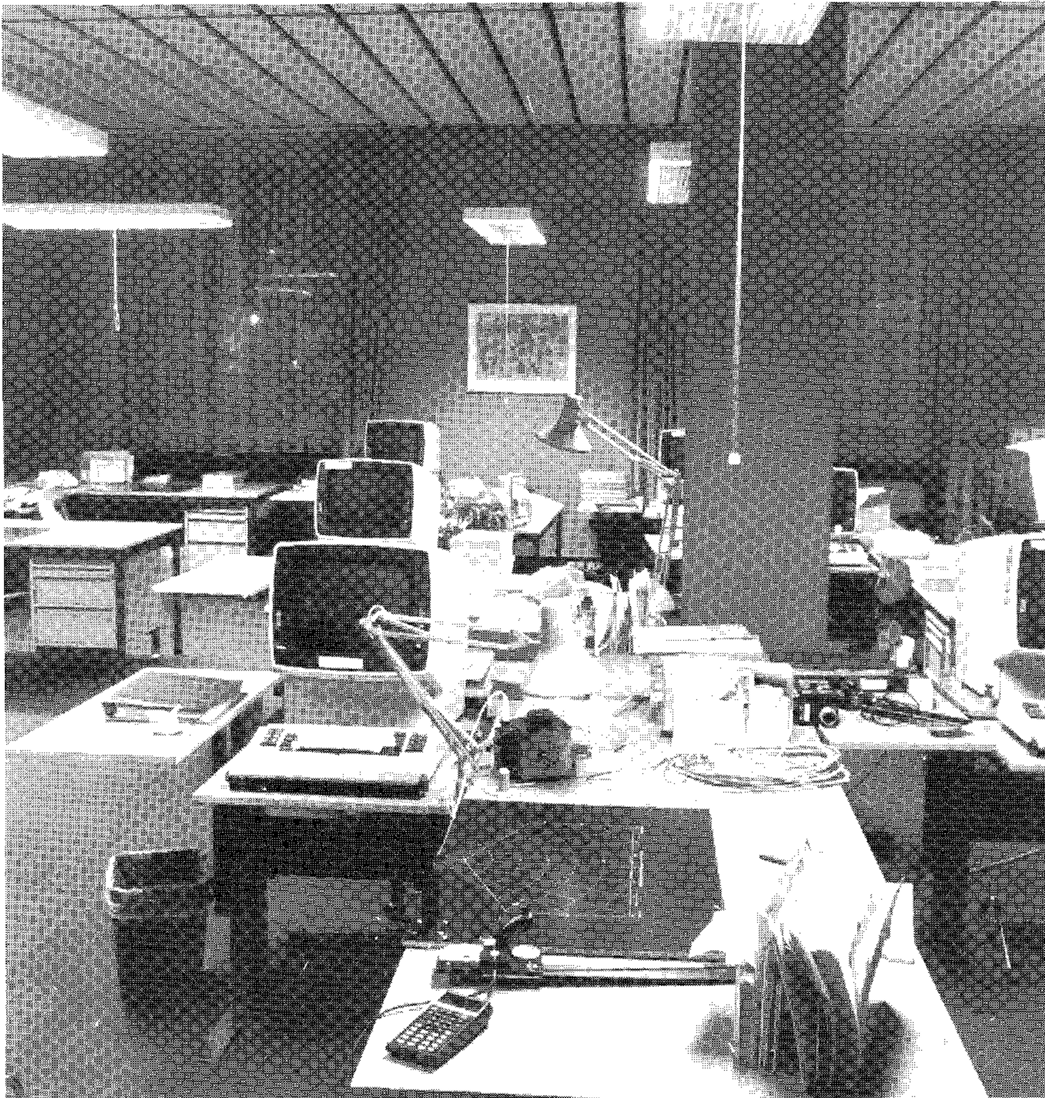
Fig. 23. An example of luminaires with low luminance louvers enabling the effects of reflections and glare on the screens to be avoided. On the other hand, the luminaires are too widely spaced to give a good contrast rendering on the desks: a localised lighting at each workplace is necessary.
